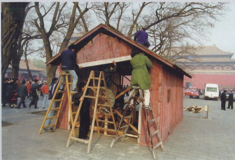
A crew in Beijing, China, erects a replica of "the garage," HP's first facility, before filming a television commercial. The garage is the focal point of HP's $200 million branding campaign.
